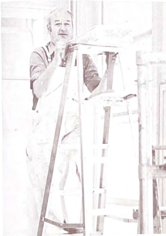
DESCENDING FROM his perch after a hard day's work is painter Tom Brown. Tom and partner Marcel Olivier are currently working on the classrooms of the first floor of the Classical Building. (Photo by Clements)
